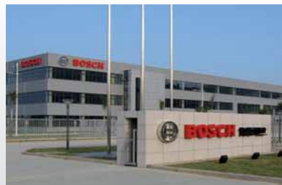
Manufacturing in Zhuhai, China
