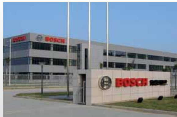
Manufacturing in Zhuhai, China
